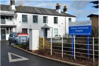
Primary Care Centre
